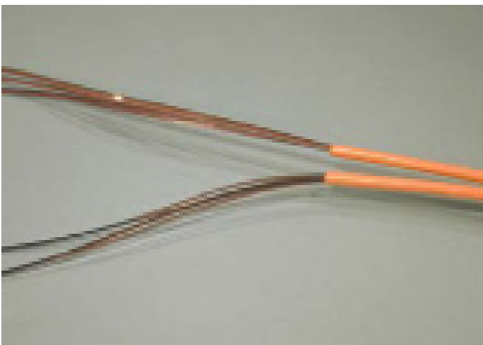
E. When all buffer tubes are cut open, fold the bare fibre ribbons and feed into the closure.
